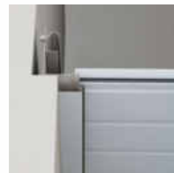
Installation behind the opening – fascia panel behind the opening
